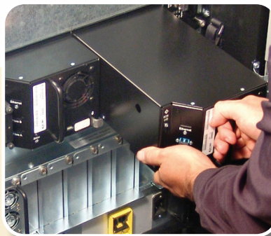
Tape Drive Replacement
